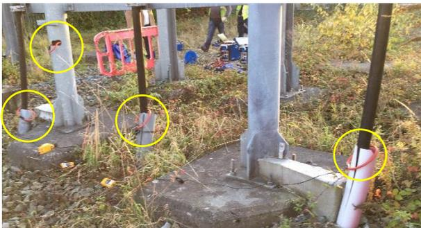
Figure 14: Primary measurement of  $I_p$  with 4 Rogowski coils
